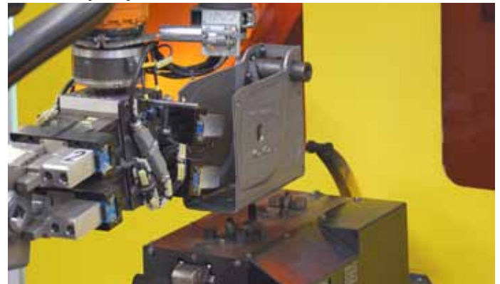
Photo 2: The handling robots load and unload the welding cells fully automatically.
