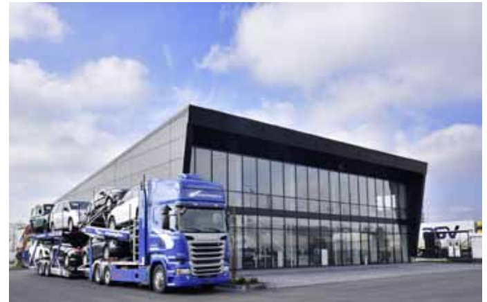
Photo 6: Example reference - a commercial building from Hörmann.
